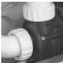
Vent air by slightly opening pump unions.
